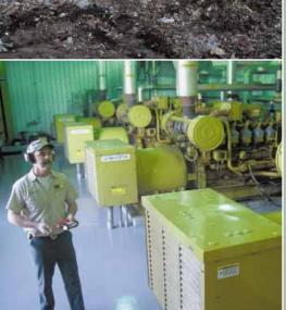
Waste Management and the Omaha Public Power District are working to turn waste into watts with a new methane gas plant at Douglas County Recycling and Disposal Facility. The \$4 million, 3.2-megawatt power plant is fueled by methane gas produced by the Douglas County Landfill, where the plant is sited.
